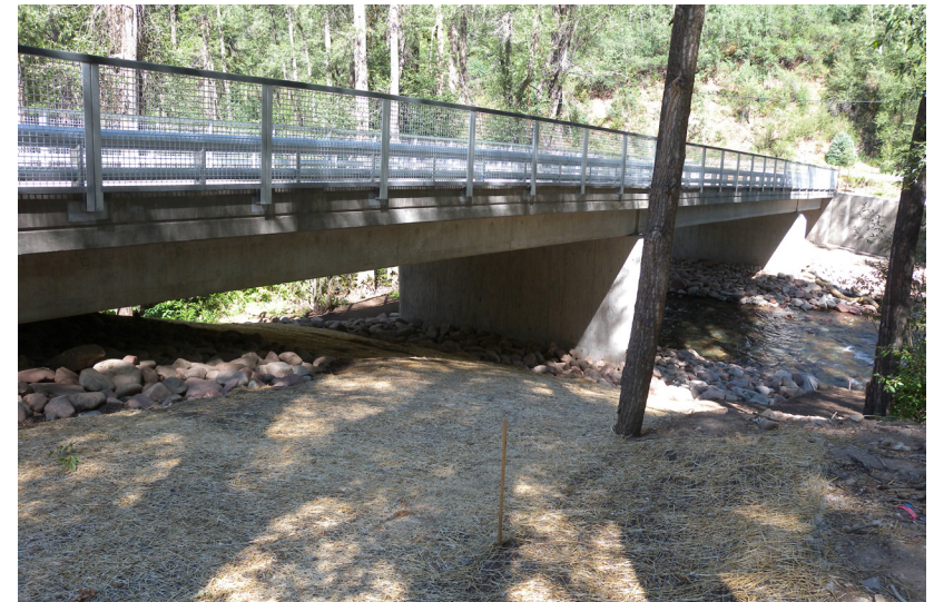
Figure 2.u: A combination of river rock rip rap and reseeding protected by erosion control blankets are used in the streambanks. These are examples of heights steps, transitions and ends. The top left angular, irregular pattern should be avoided.
