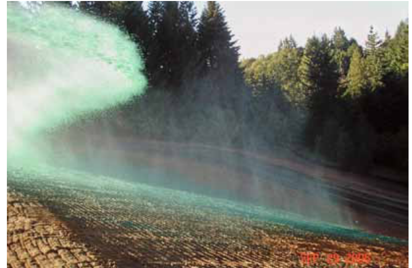
Figure 2.zzi: Hydro-mulching is a technique to seed large areas of land.
