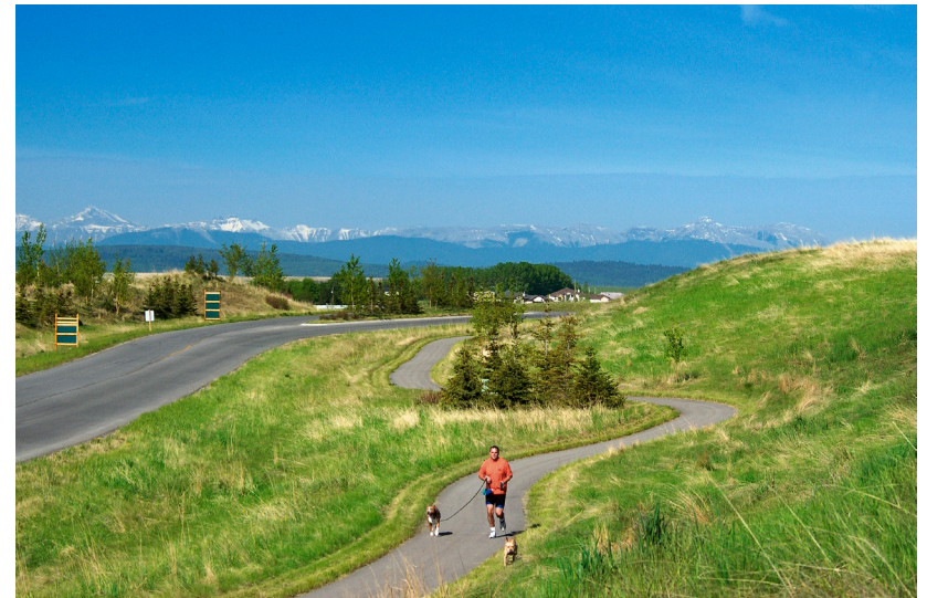
Figure 4.b: Transportation alignments should consider and provide for adjacent communities as in this example.
