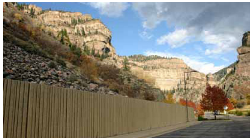
Figure 3.zp: The color selection for this wall is based on the natural tones of the cliffs.
