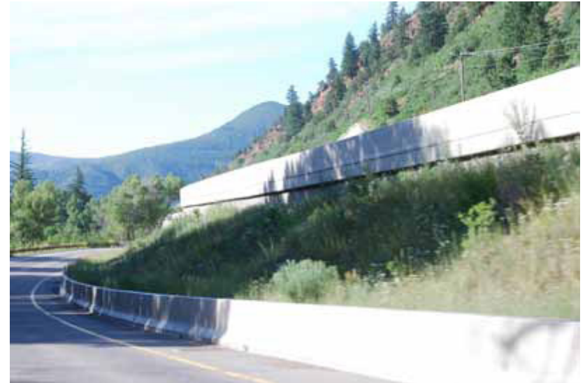
Figure 3.zh: Utilize continuous concrete barriers.
