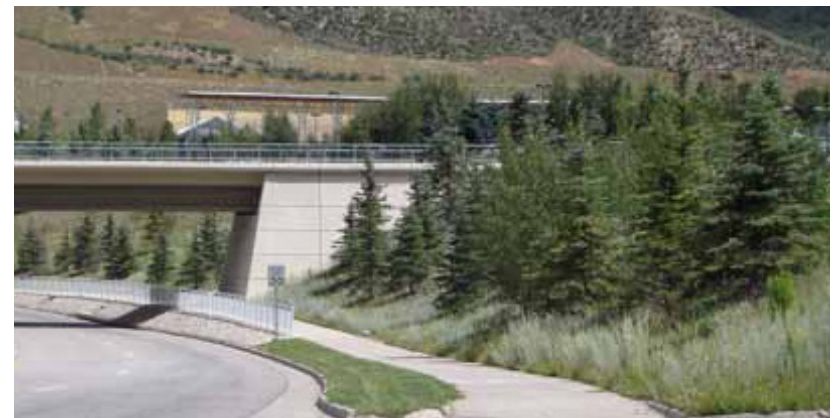
Figure 3.o: Use vertical abutment design to limit slope paving and provide space for planting.
