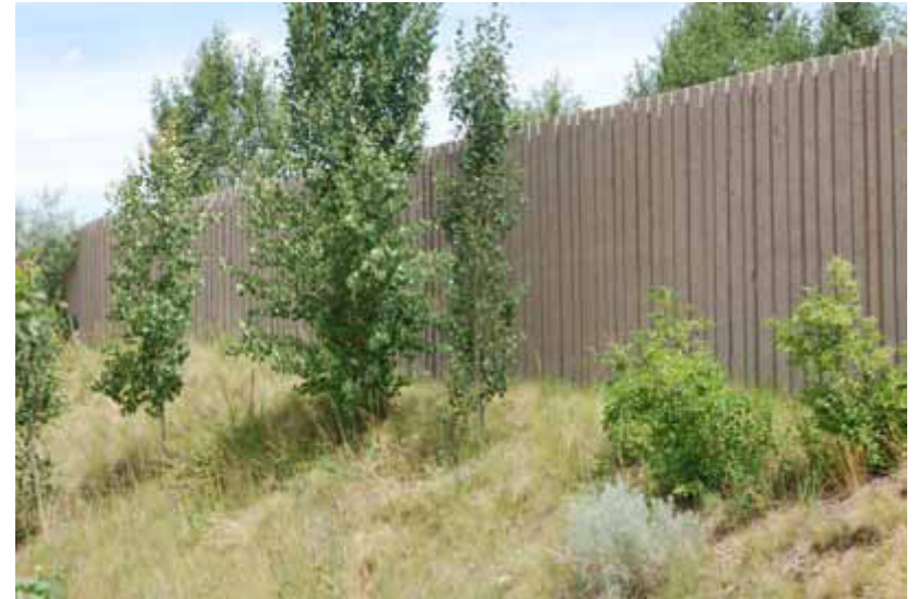
Figure 3.zb: The use of grading allows for reduction in height of the wall and also for landscape planting.
