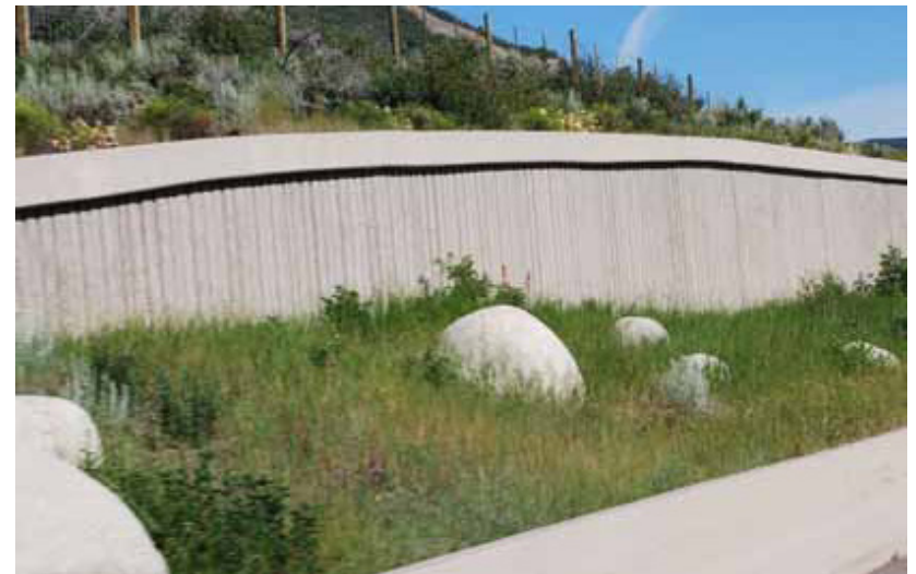
Figure 2.zq: In the highway environment, hardy grasses and shrubs are required. Boulders add interest to the planting.
