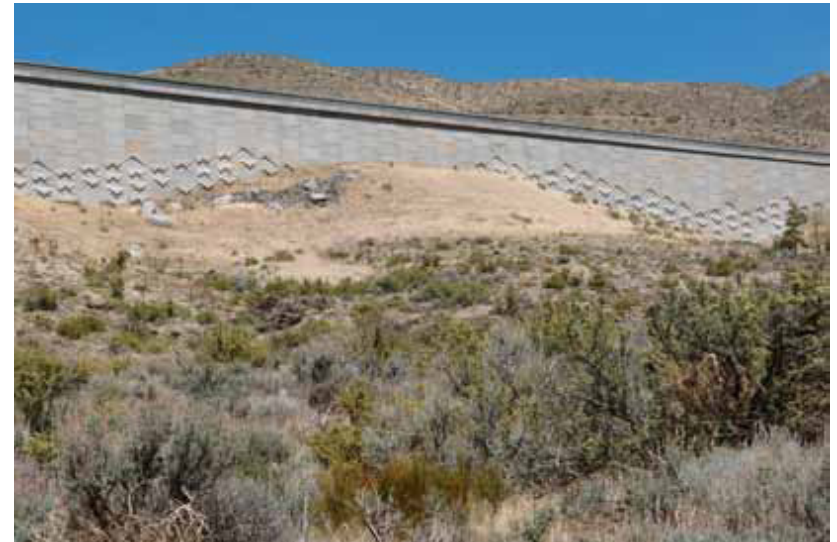
Figure 3.zu: Transportation art may be incorporated directly into the highway design like the patterns in this retaining wall.
