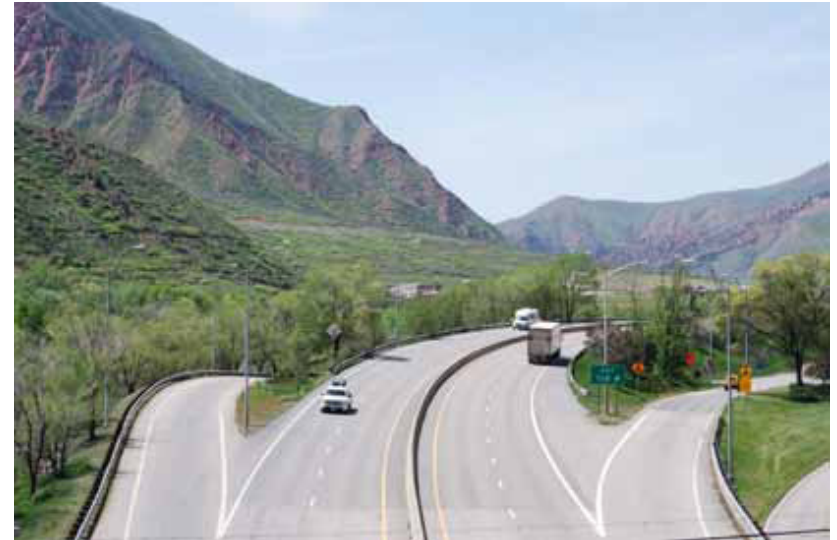
Figure 3.g: This divided highway utilizes narrower lane widths and vegetated medians to respond to the landscape context.
