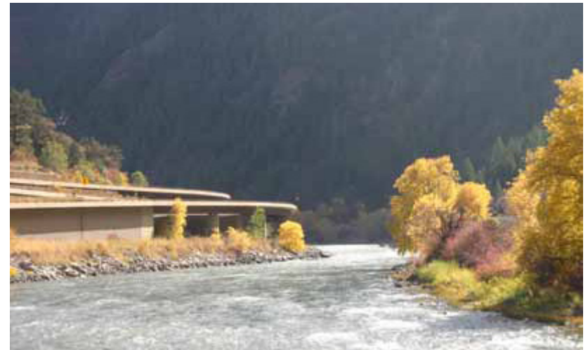
Figure 3.h: This elevated highway is a sensitive response to preserving the river and riparian environment.
