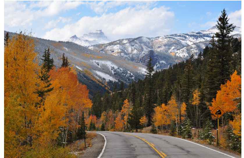
Figure 1.b: This highway near Durango has been designed from a contextual perspective.
