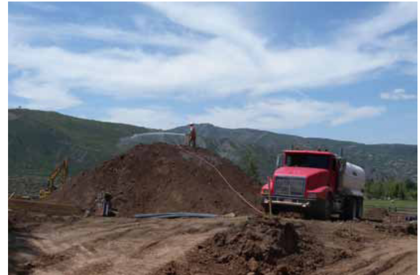
Figure 2.zzh: Topsoil is stockpiled on site and watered to minimize dust.
