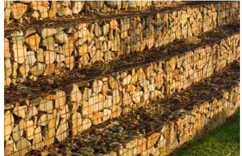
Figure 2.zf: Well constructed rock gabions.
