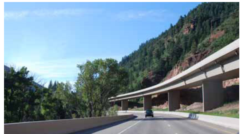
Figure 3.e: The elevated structure of Highway 82 minimizes impacts to the steep rocky topographic conditions.
