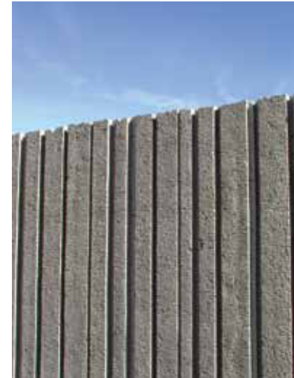
Figure 3.zd: Vertical patterning is useful as it conceals vertical joints.
