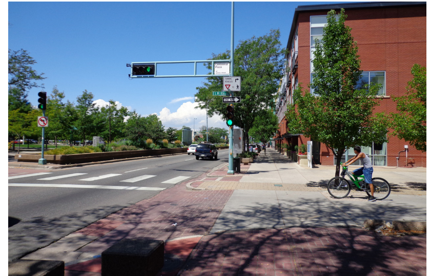
Figure 4.i: Use of different paving materials, pedestrian crossing markings and traffic lights promote traffic calming.
