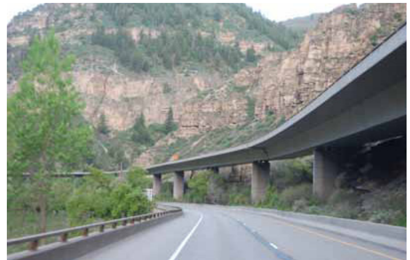
Figure 3.l: This is an example of compatible proportions and consistent treatment of structural components and finishes.
