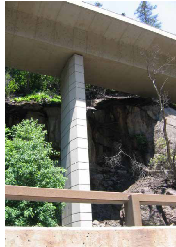
Figure 3.s: The visual prominence of the pier is reduced by using simplified surface treatment.
