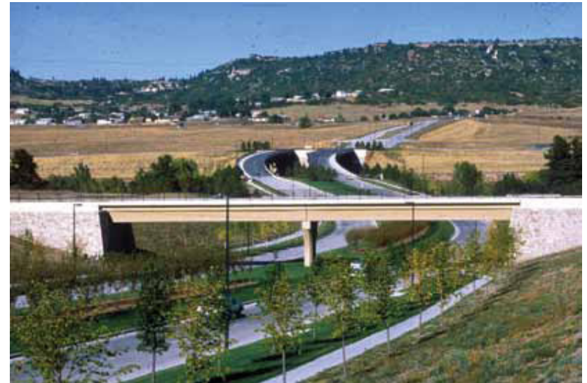
Figure 3.k: This bridge illustrates thoughtful consideration of the design components.
