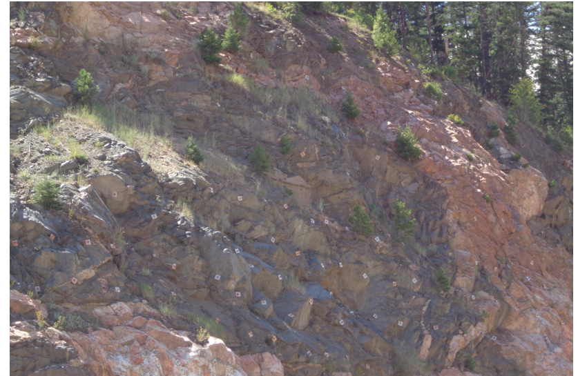
Figure 2.s: Soil nail techniques are used for stabilizing rock faces.
