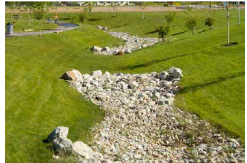
Figure 2.zi: Riprap lined drainage swales provide stormwater treatment in an urban area.
