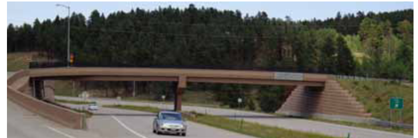
Figure 3.n: Two spans cause a split composition but appear appropriate due to the highway configuration and the median.
