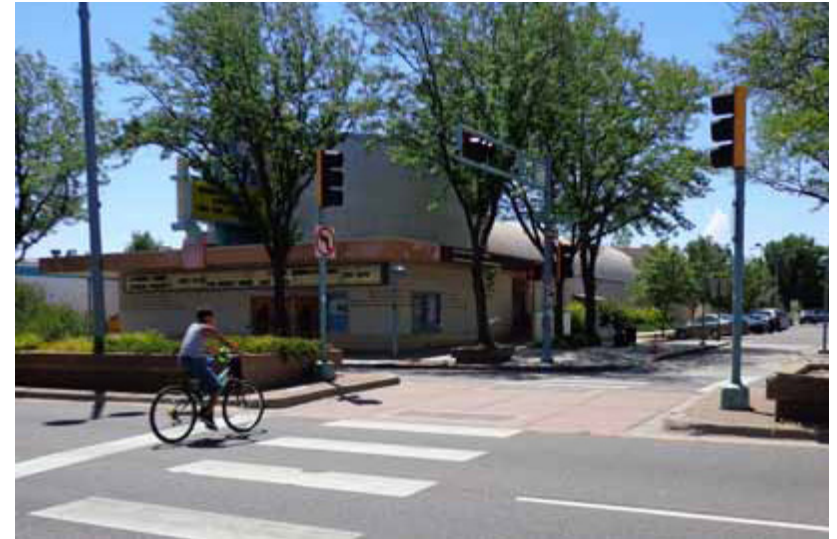
Figure 4.s: This road crossing is designed to accommodate bicyclists and wheelchairs with the on-grade median crossing.
