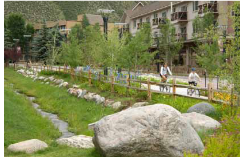
Figure 4.x: A shared use path that is separated from the roadway, adjacent to a landscaped storm water system.
