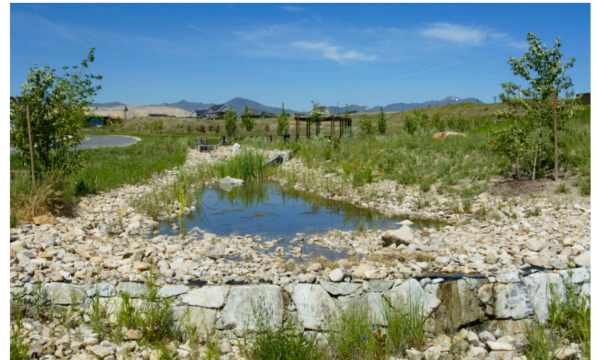
Figure 2.d: This pond serves to detain stormwater and create habitat.
