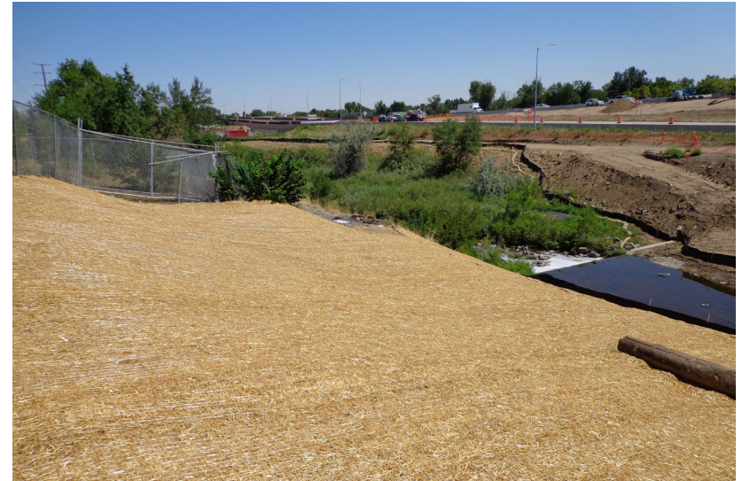
Figure 2.v: A variety of techniques are used in this urban setting. They include chain link fencing for site protection, straw erosion control matting and black silt fencing to trap sediments.
