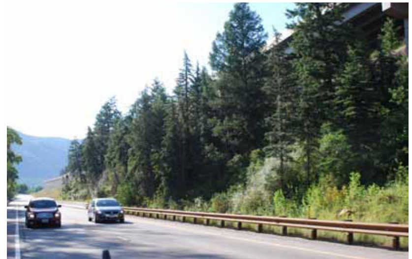
Figure 2.zl: This separated highway provides protection of existing trees.
