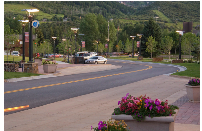
Figure 4.e: When highways become Main Streets, the character changes to be more pedestrian friendly.
