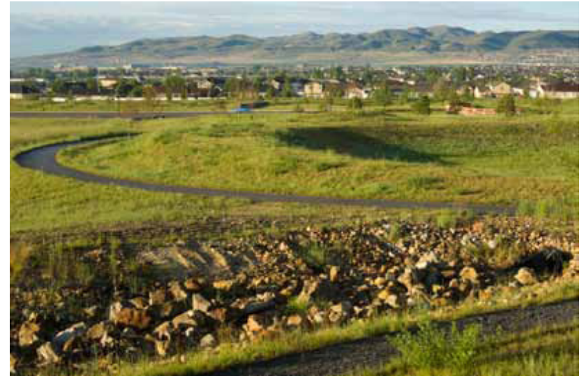
Figure 4.ze: This grading for storm water detention uses rounded and naturalized slopes, in addition to the naturalized channel with riprap.
