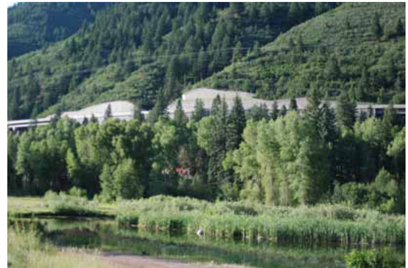
Figure 2.zg: The riparian valley adjacent to the stream is preserved since the highway is located upslope.
