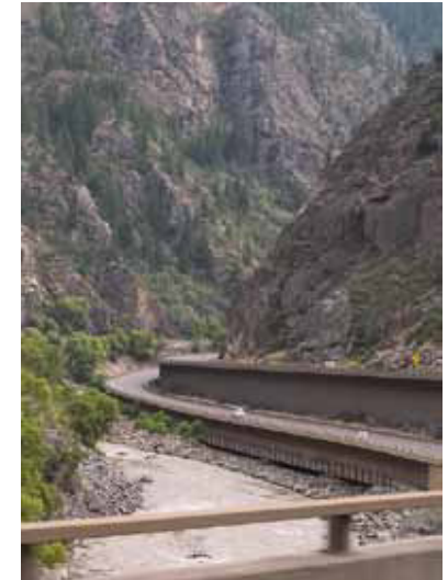
Figure 3.d: This interstate highway was located with careful consideration of the landform and topography of Glenwood Canyon.
