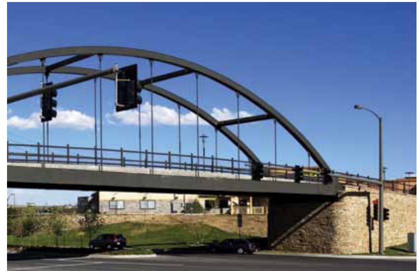
Figure 3.u: Pedestrian bridges may be smaller scaled and more decorative than highway bridges.
