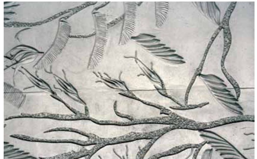
Figure 3.z: This twig pattern in concrete is simple and allows variety through placement in different orientations.
