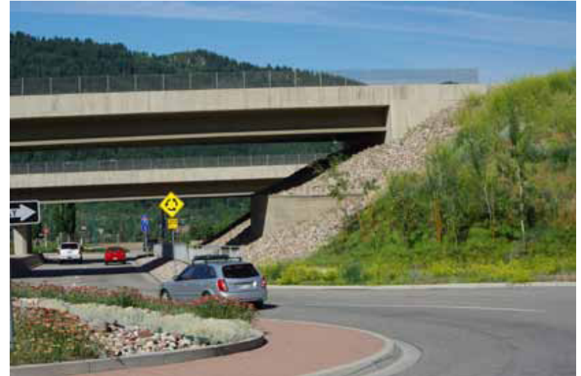
Figure 3.q: The heights of the abutments are reduced and combined with a sloping face.
