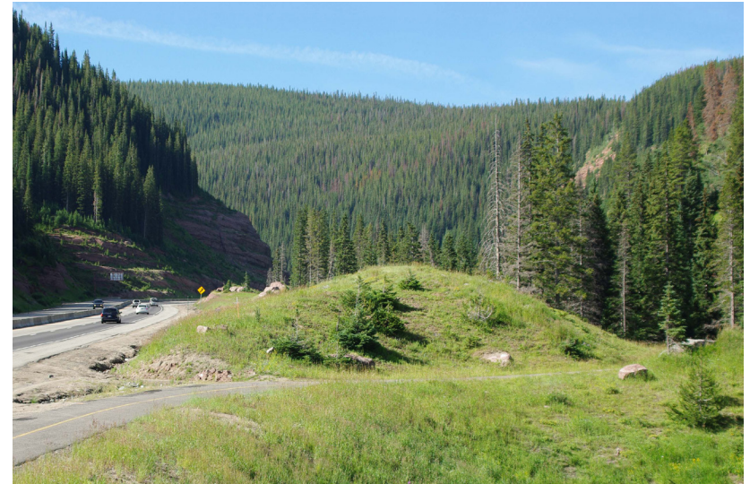
Figure 2.o: These slopes have been rounded to provide a stable area for revegetation.
